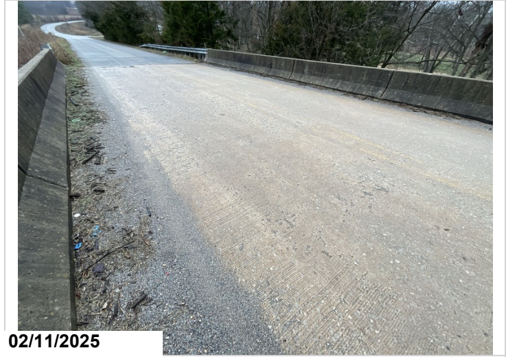
Span 1, Right Lane: Moderate abrasion.
