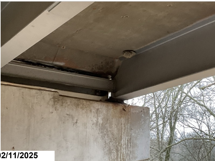
Spans 1 - 3, Bents 1 & 2, Girders 1 & 4: Moderate active corrosion with pack rust.
