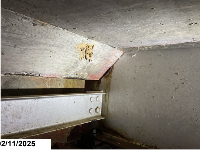
Abutment 1 & 2, Girders 1 & 4: Moderate active corrosion with flaking rust.
