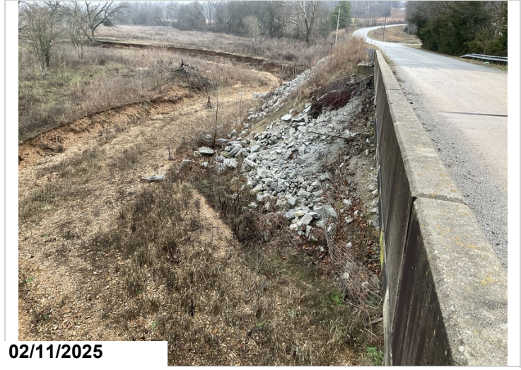
Large rock has been added to the channel.
