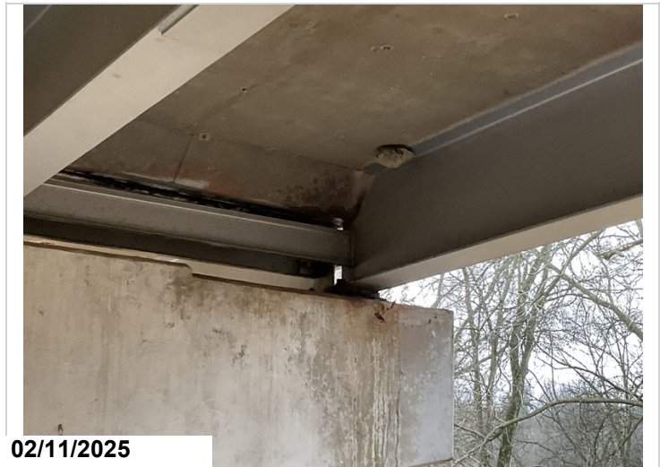
Spans 1 - 3, Bents 1 & 2, Girders 1 & 4: Moderate active corrosion with flaking rust.
