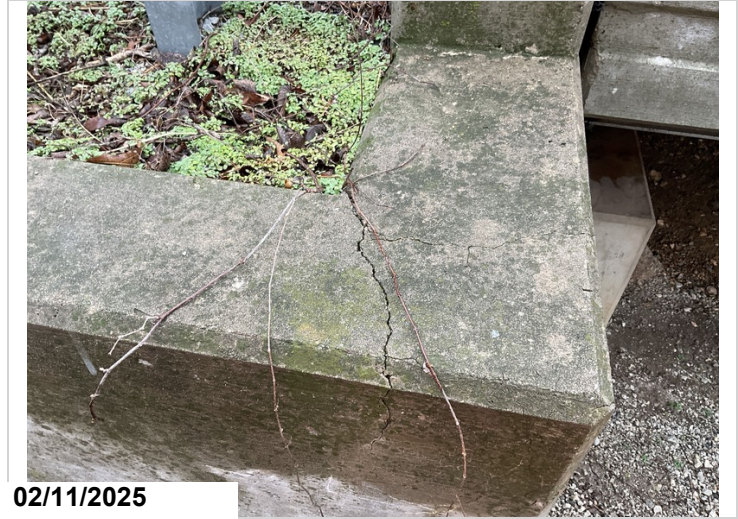
Abutment 2, Left: Cracking.
