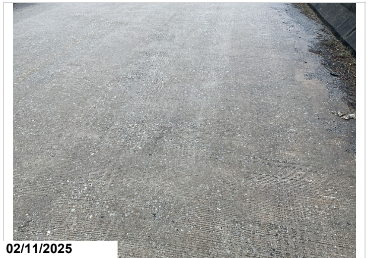
Spans 1 - 3: Minor abrasion.
