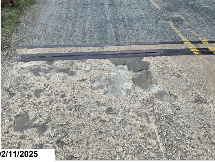
Span 1, Right: Spalling.
