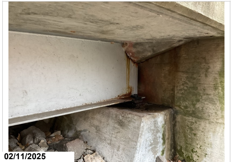
Abutment 1 & 2, Girders 1 - 4: Active corrosion with pack rust.
